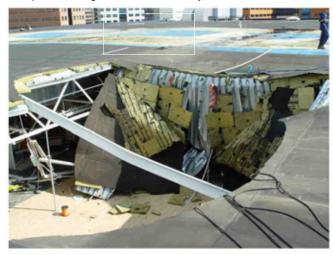
The main problem was that driving rain apparently washed over edges that where designed to hold the water. This is the movitivation for the key research question: Can we simulate the height of the water near the edges of an inclined roof during heavy rainfall and wind gusts?
