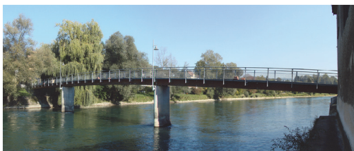
Figure 1. Photo of timber bridge.
